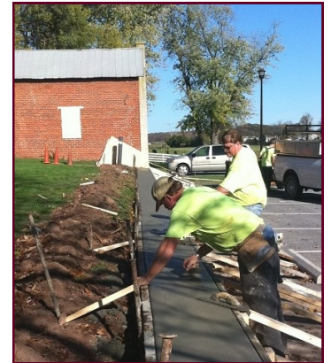
Don and Doug Lamb trowel the concrete for a smooth finish.
