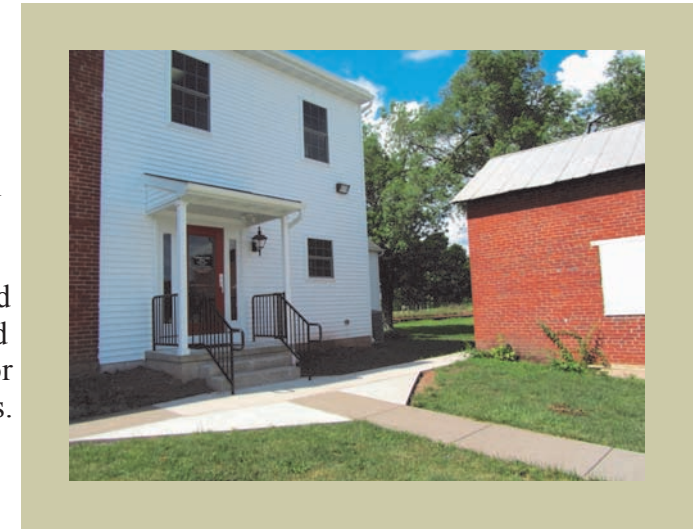
Tina Tatnall is planning a serenity flower garden in the area between the walkway and the brick shed.
